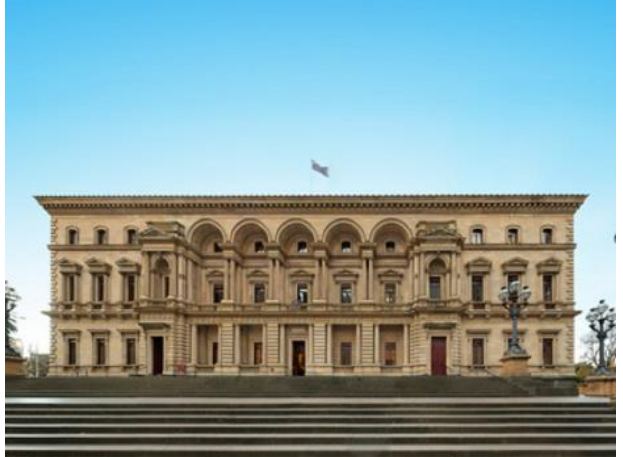
Old Treasury Building
